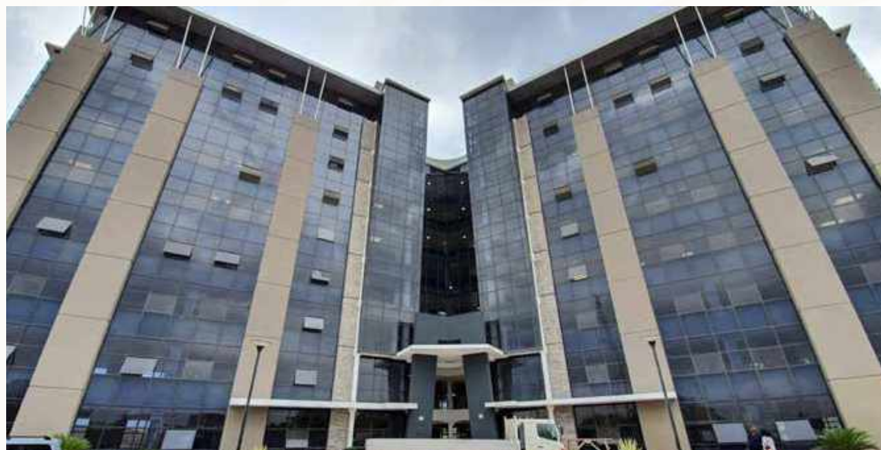
Above: ZEP-RE Business Park in Lusaka, Zambia
